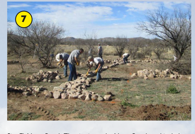
Site 7) Noon Ranch: The site is on the Noon Ranch, and includes watershed restoration work installed in 2016 using rock erosion control structures in the uplands of the North Branch of the Arivaca Creek and the adjacent Sacaton grassland. There is also a burn plan for this site, which is being worked on in conjunction with the Buenos Aires National Wildlife Refuge.
