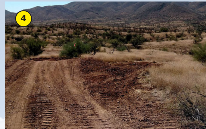
Site 4) Rancho Seco: The site, on Pima County owned Rancho Seco, includes watershed restoration work using rock structures and road drains, installed spring and fall 2016. Installing rolling dips, like the one in the photo, as road drains waters a quarter to a half an acre of land using water harvested off of the road.
