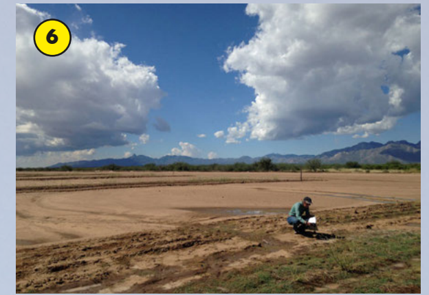
Site 6) Northern Altar Wash Area: The site is on the Pima County owned 98 Ranch. The restoration work installed in 2016 is designed to restore grassland vegetation to retired, barren agricultural fields by using low berms to mimic the effect of watering and drying patterns in the historic Altar Wash floodplain.
