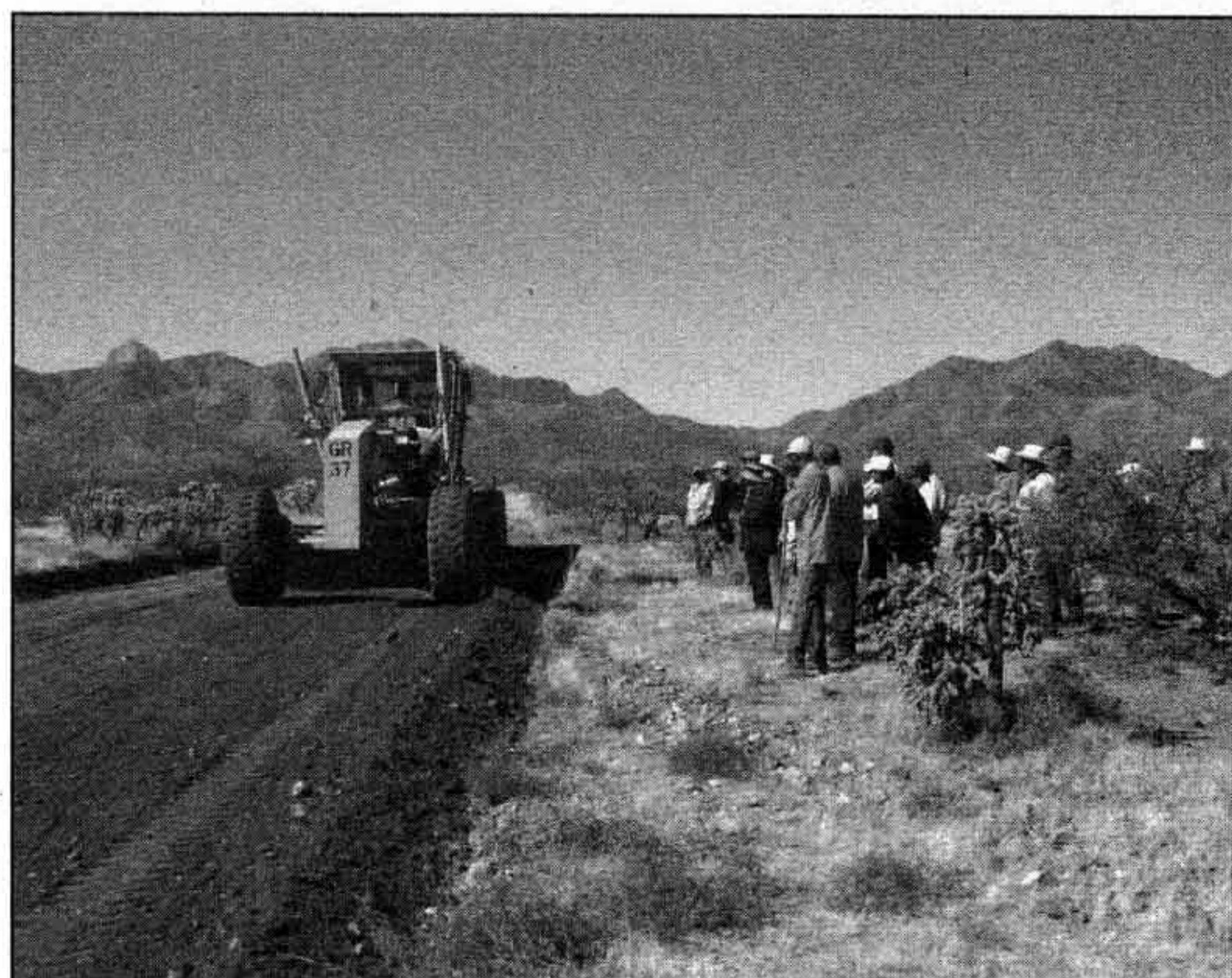
Left ... The road aspect of Zeedyk’s work focuses on teaching people about draining roads properly. Well drained roads are easier to maintain and put water back on the land where it belongs.
